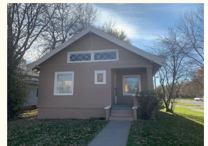
Our Billings Office after the renovations
